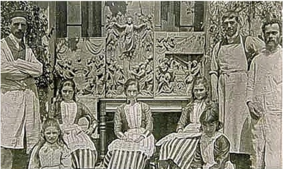
The Pinwill Sisters and Edmund Sedding with the reredos panels prior to installation
